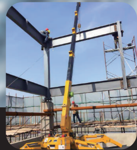
Steel structure installation
